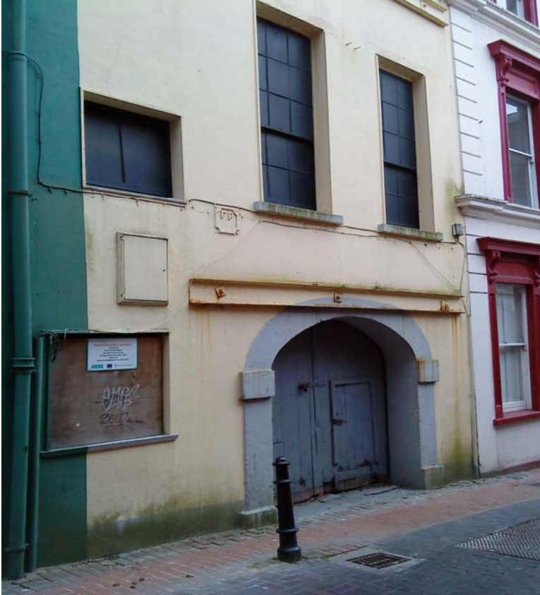
Building 4: 7 Henrietta Street, Waterford.
